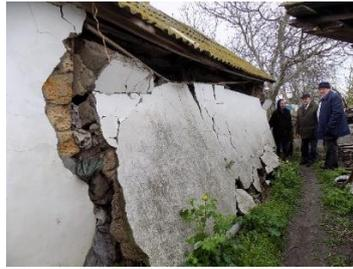
Figure 2 Destruction of residential structures due to flooding (Urban-type settlement Nova Maiachka, Kherson region, 2019).
